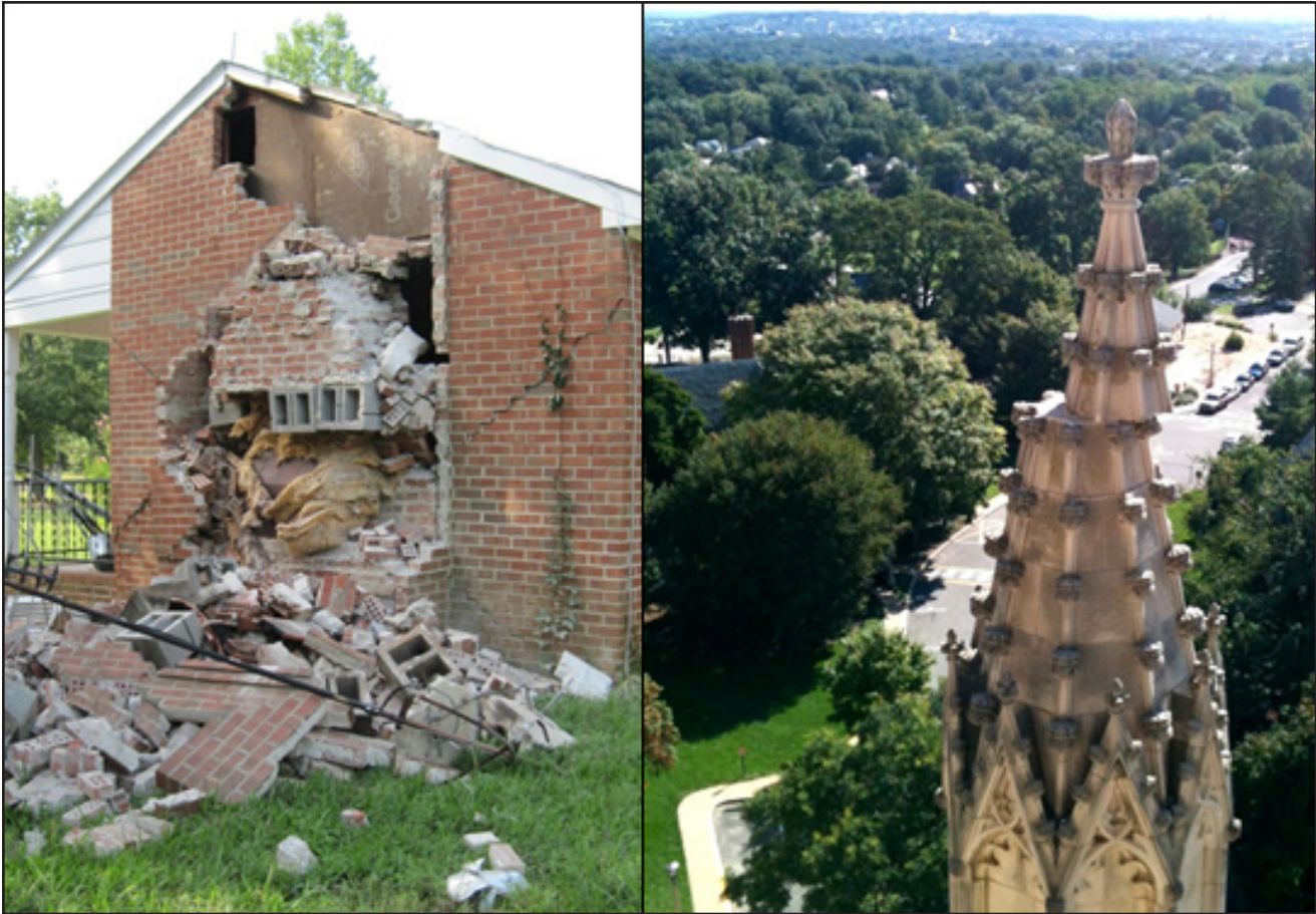
Figure 24. Property damage near the 2011 Mineral earthquake epicenter (left) and the steeple of the National Cathedral in Washington, D.C. that was displaced (right). Photos by Francis Ashland, U.S. Geological Survey.
